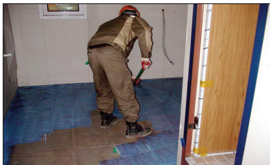
Priming steel deck
